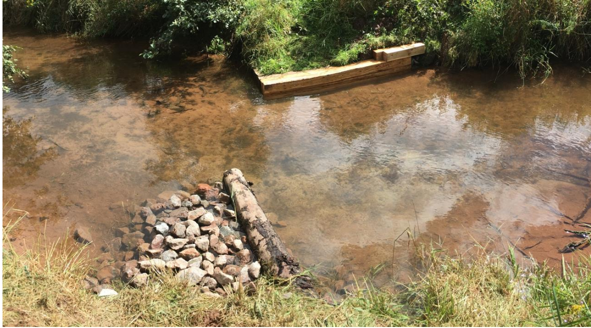
Figure 6. The upstream log wing (near) and log crib (far) deflectors built in 2017, pictured after the 2020 enhancements.
