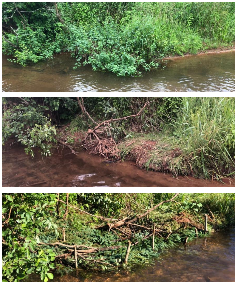
Figure 8. A cluster of bittersweet nightshade, an invasive species (top). Exposed sediment after the nightshade was removed (middle). The finished brush mat with dogwood plantings (bottom).
