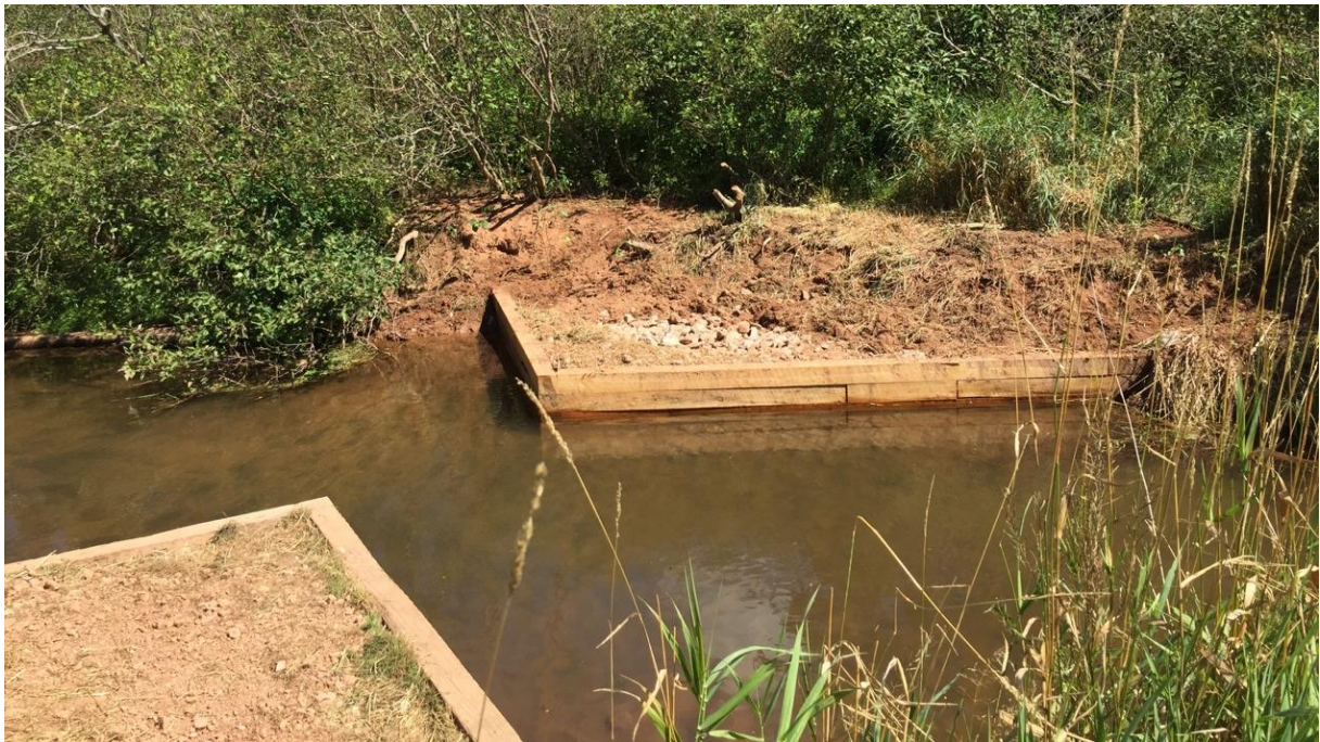
Figure 5. The downstream 2017 (near) and 2020 (far) log crib deflectors.
