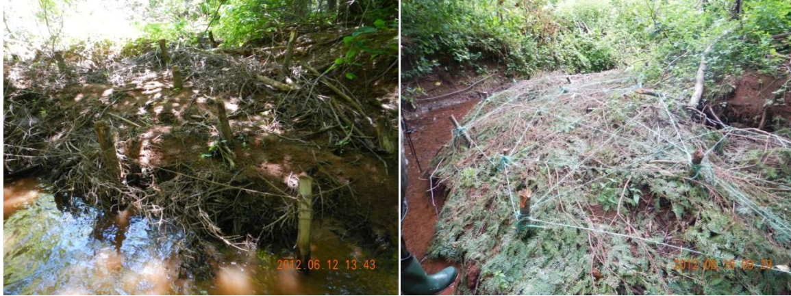
Left: Brush mat built in 2011. The silt has been trapped between the thick layers of soft wood branches. Right: A new brush mat completed in 2012 that will collect silt and will look like the picture on the left after the high waters in spring and fall.
