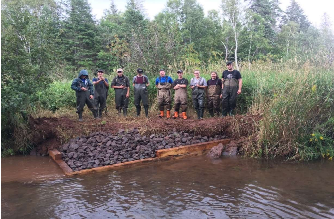
Figure 7: Central Queens Wildlife Federation, Bedeque Bay Environmental Management Association and Wheatley River Improvement Group with Finished Log Crib Deflector.
