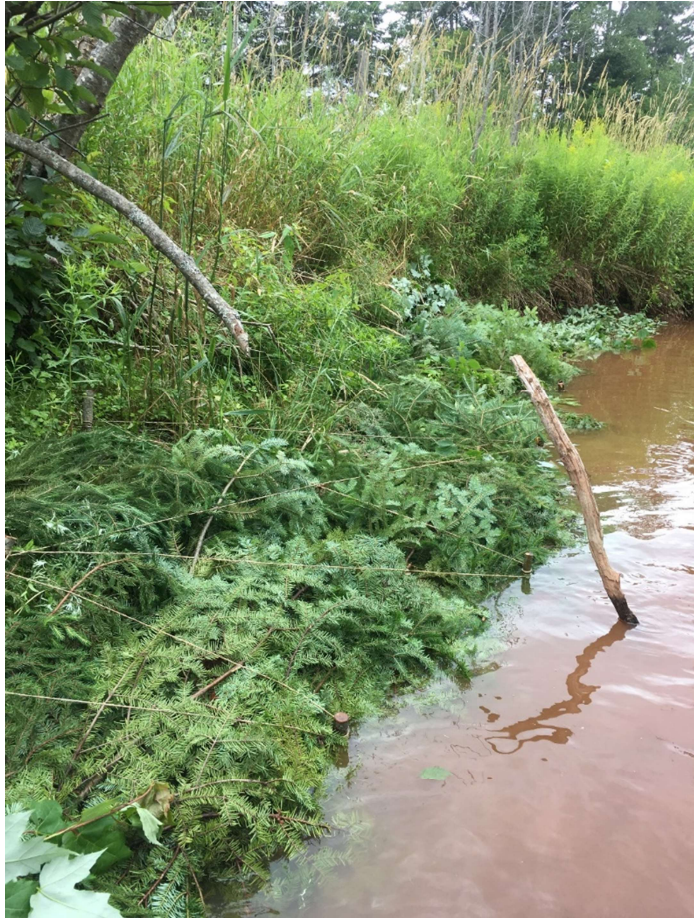
Figure 3: Brushmat Installed on Property #992347 on Crooked Creek Main Branch in old Beaver meadow to Help Stabilize Stream Banks.
