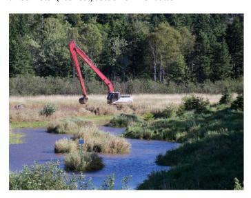
River depth here has been improved from 12-18 inches to 6 or 7 feet and will now serve as safe habitat for aquatic species and likely as a spawning area for brook trout for many years. The area will also serve as a catchment site for sediment flowing downstream, allowing silt to settle out here before it enters the much deeper pond and the river below.
