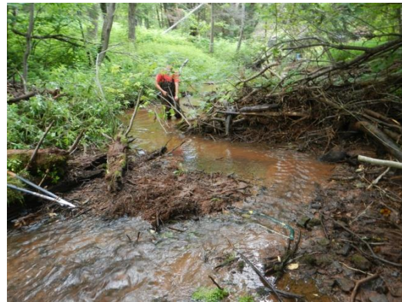
Figure 3 & Figure 4. An example of stream restoration: before and after pictures taken of stream cleaning on Parker Cross Road. There was immediate improvement to stream flow, and movement of sediment from stream bottom.
