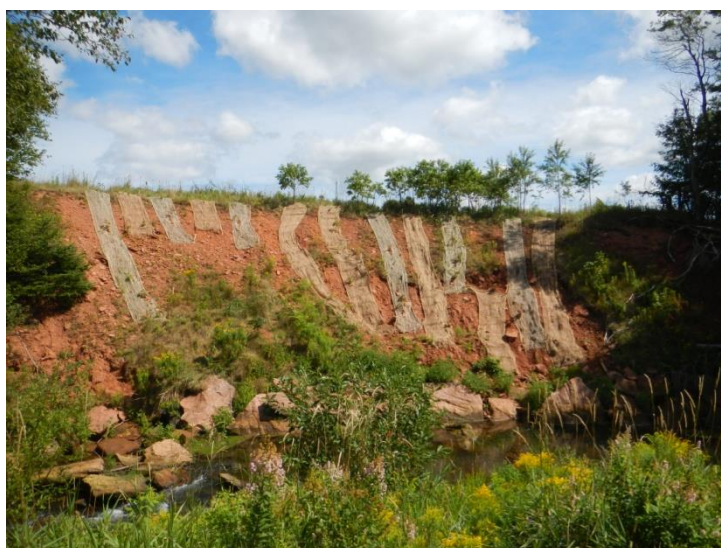
Figure 7. Jute matting installed to reduce erosion on the slope below Rackham's Pond, and encourage plant growth.
