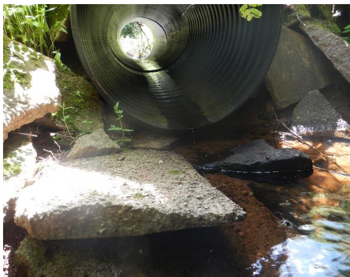
Figure 6. Hung culvert with low flow, an obvious barrier to fish passage.
