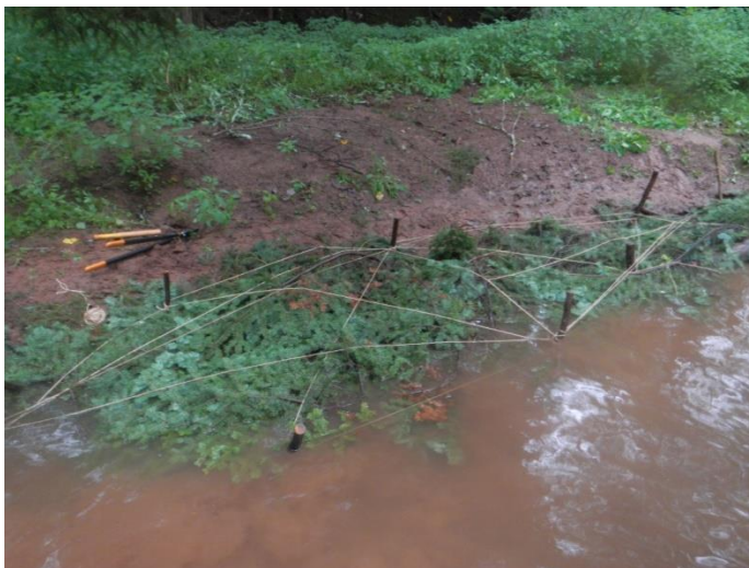
Figure 5. Brush mat made of spruce boughs and anchored with alder stakes and twine, Millboro Road.
