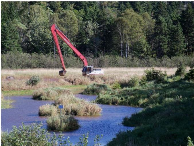
River depth here has been improved from 12-18 inches to 6 or 7 feet and will now serve as safe habitat for aquatic species and likely as a spawning area for brook trout for many years. The area will also serve as a catchment site for sediment flowing downstream, allowing silt to settle out here before it enters the much deeper pond and the river below.
